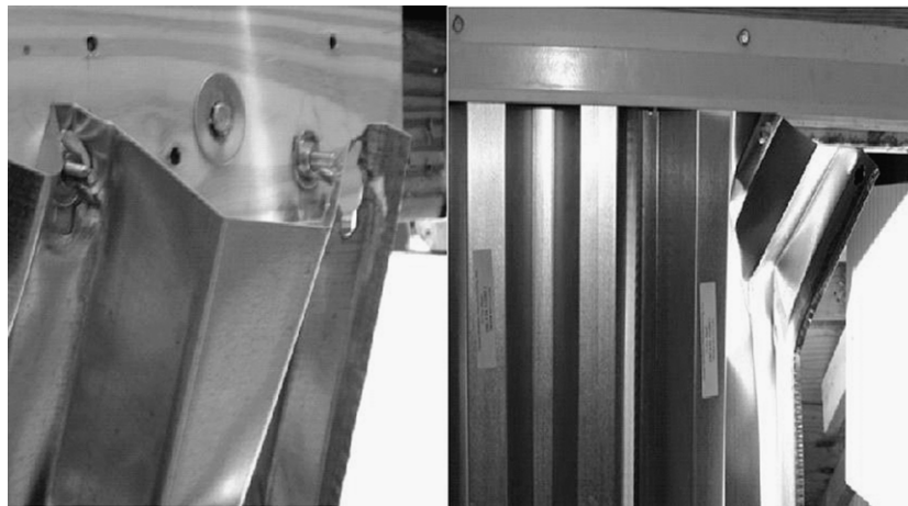
Fig. 12. Examples of direct mount tear (left) and track mount pull-out (right).
